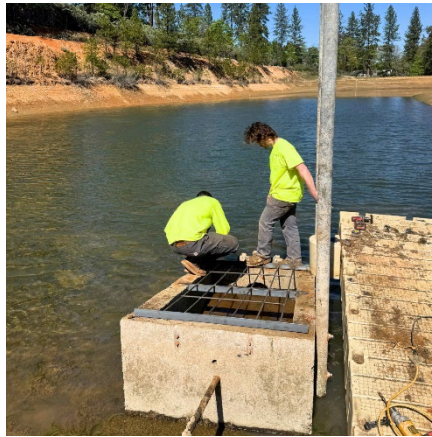
RESERVOIR OUTLET INSPECTION
